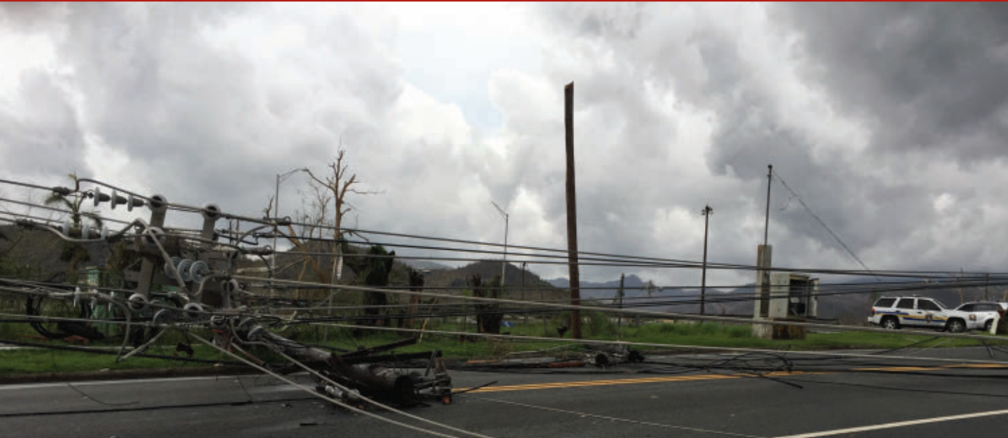
Fallen trees and electrical wires blocking the expressway entrance
